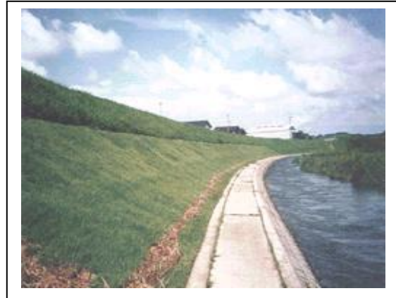
Fig. 10 : Final view of layered Green growing concrete
